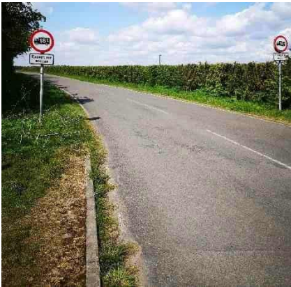
Figure 2-5: High Ditch Road- Site Visit
